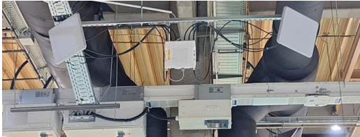
Figure 3. Installing and commissioning the second AP
