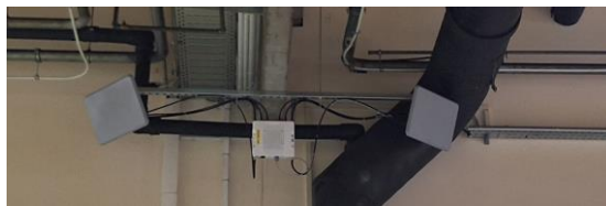
Figure 2. Installing and commissioning the first AP
